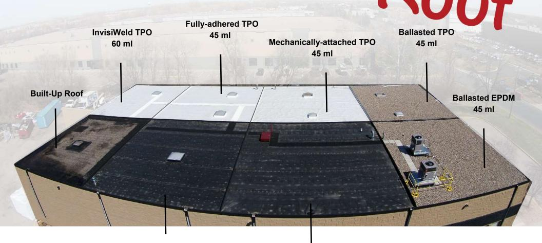
Fully-adhered EPDM 45 ml reinforced & 60 ml
